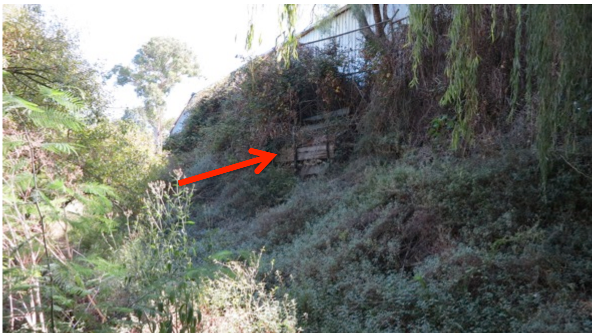
Minor retaining walls (arrowed) are evident on the south side of the Monumental Masons site and were presumably constructed to retain fill. The property boundary here is uncertain as it could be either the retaining wall or the fence line above.
