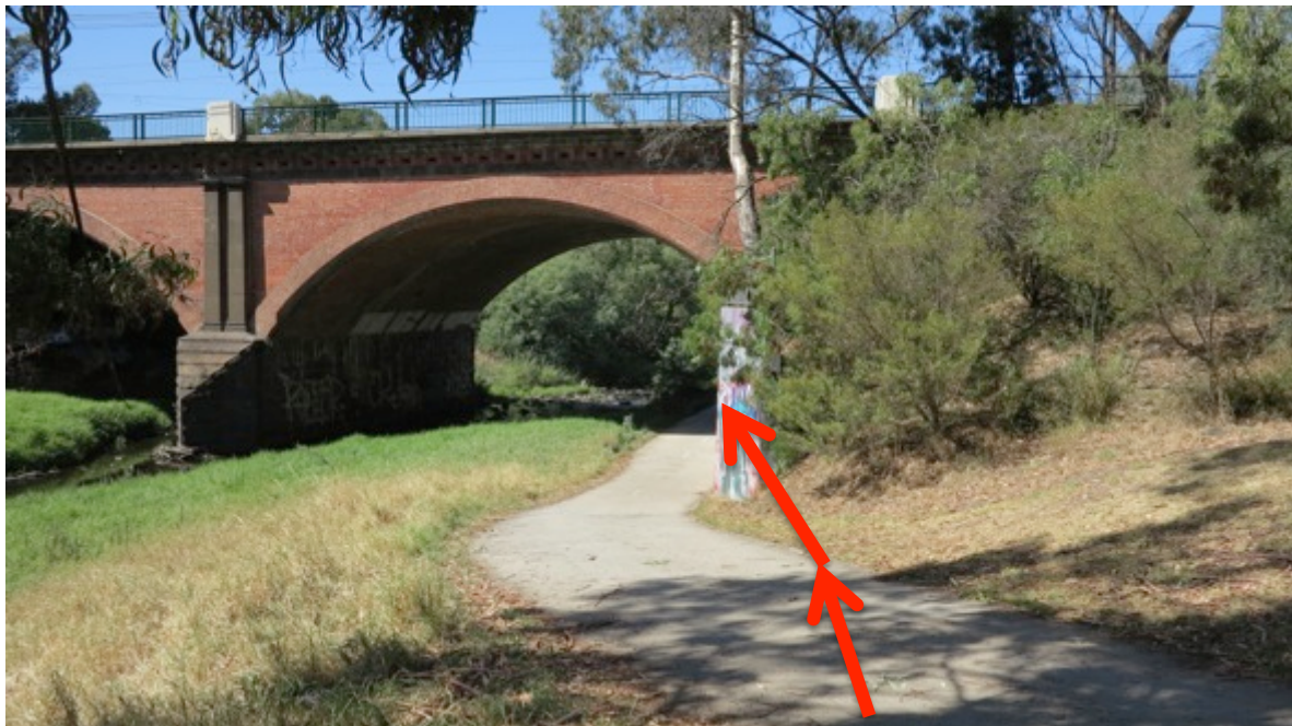
The High Street bridge underpass. The new MCT/CCT (arrowed) would be elevated on a boardwalk under the bridge. Investigations would need to ensure cross-sectional area for flood passage under the bridge was not compromised.
